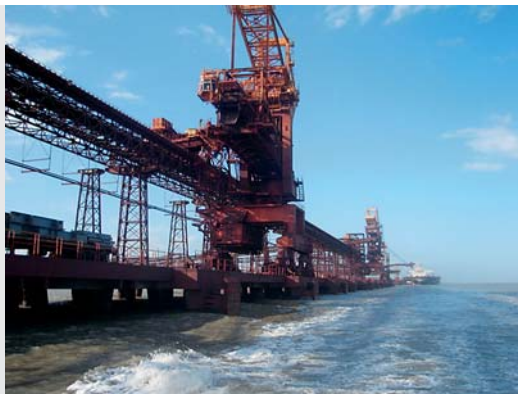
Ponta Da Madeira (Brasil) Pier III expansion with a new shiploader which started operations in September
