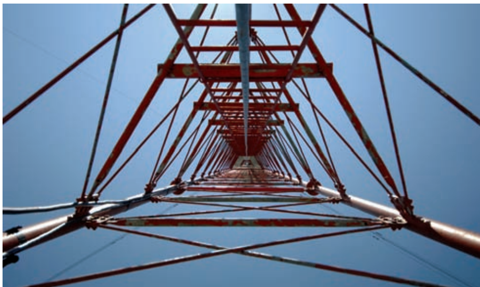
Inside one of the 625-ft towers at the Carolina Beach Loran Station - the facility's 650,000-watt radionavigational signals will cease transmission by October 2010
