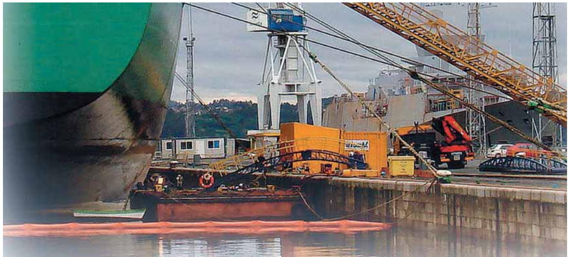
Work space established around the vessel
