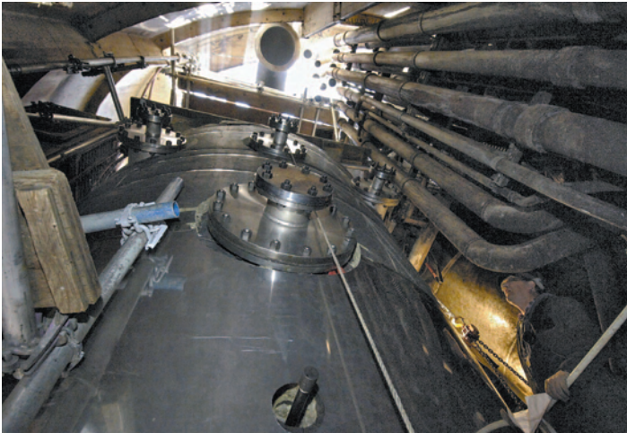
Krystallon scrubber being installed on the cruise vessel Zaandam in April 2007
